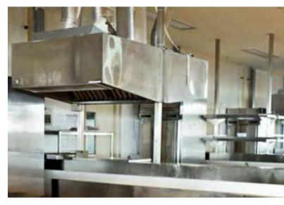
Heat exhaust hoods vent fumes from high heat cooking equipment without needing grease collected. You'd likely install heat exhaust hoods over pizza ovens and convection ovens that won't give off a significant amount of smoke, but may produce steam and excess heat.
